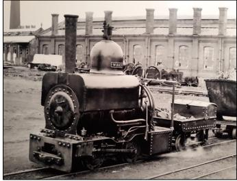
coal had outside cylinders with Hackworth valve gear.
